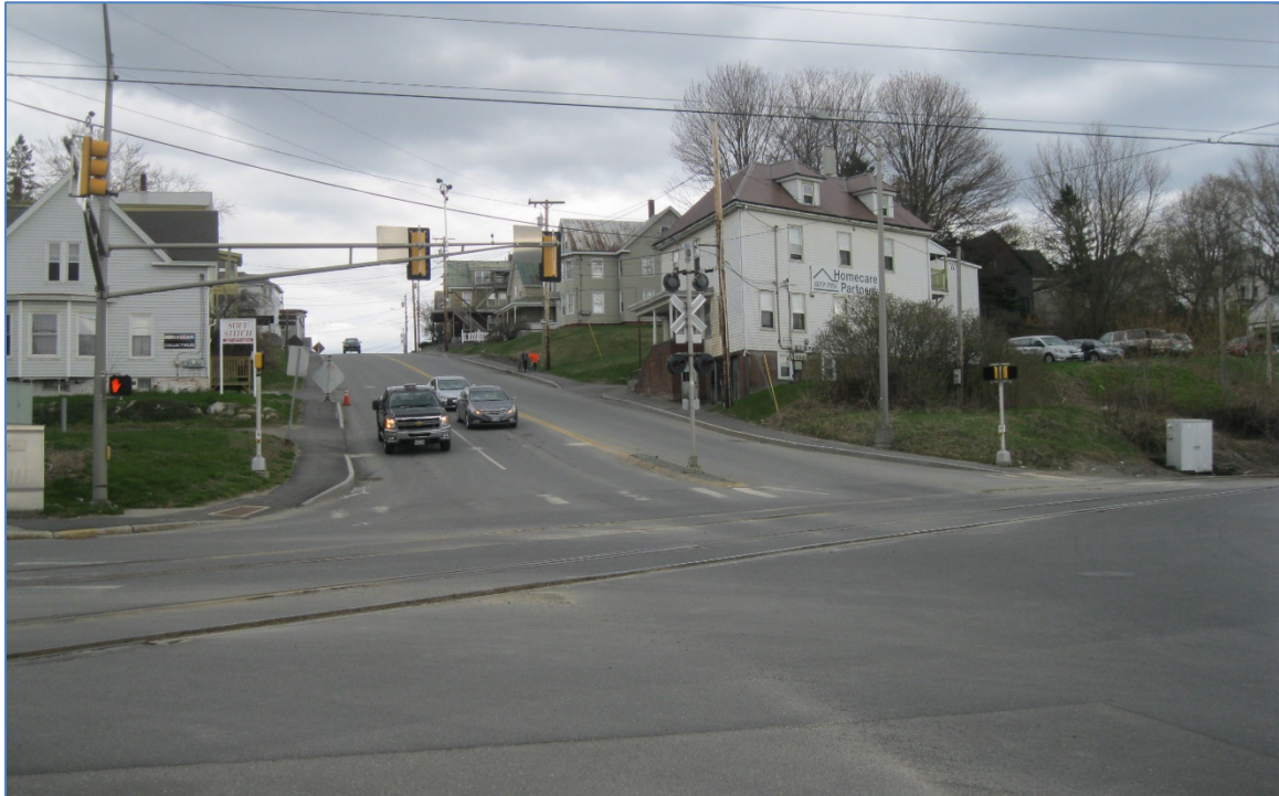
Figure 20 - Winslow Intersection Looking East
