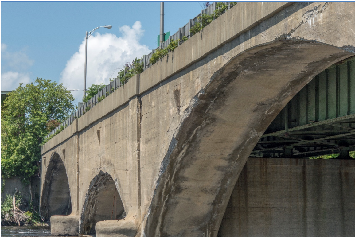
Figure 2 - Arch Looking West
