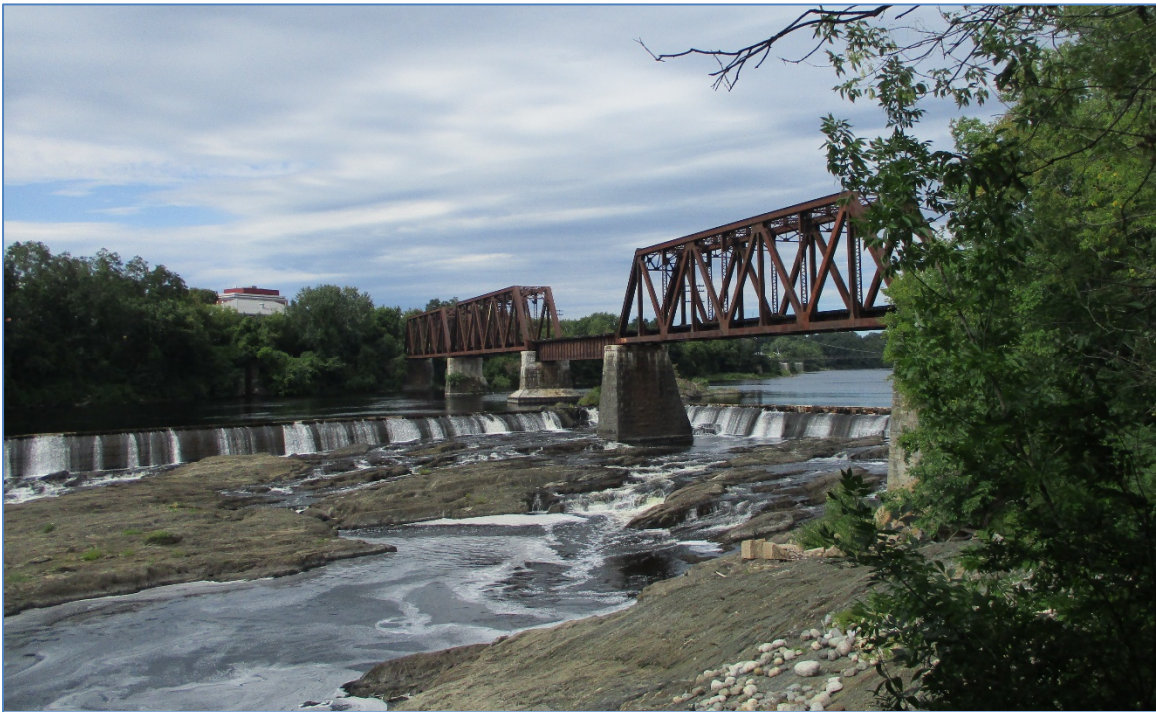
Figure 18 - Upstream Railroad Bridge Looking Northwest
