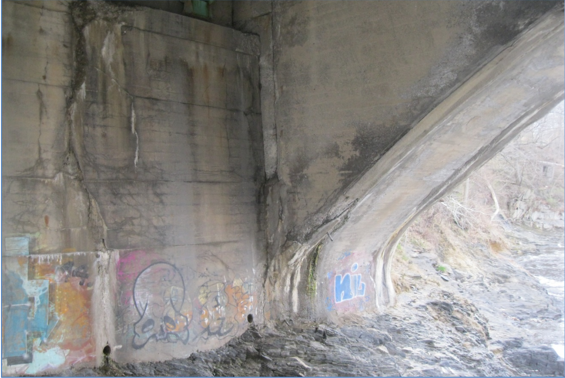
Figure 11 - East Abutment Looking Southeast
