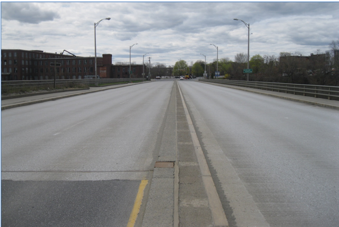
Figure 4 - Bridge Deck Looking West
