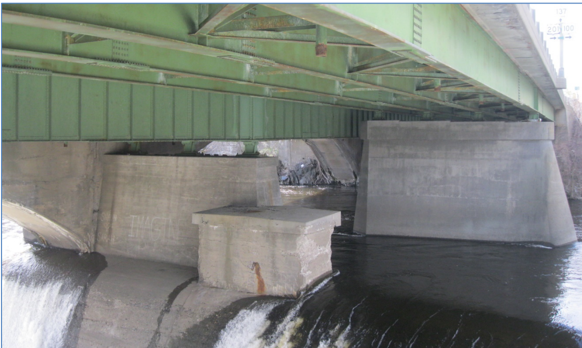
Figure 16 - West Piers, Looking West
