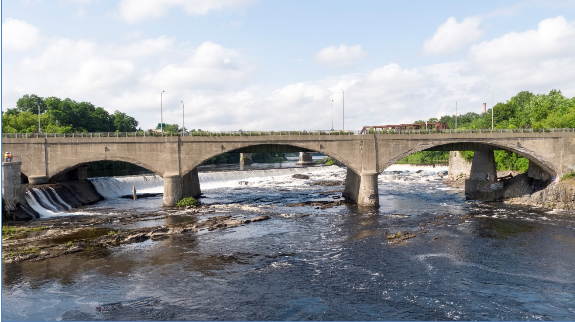
Figure 1 - Downstream Elevation of Arch
