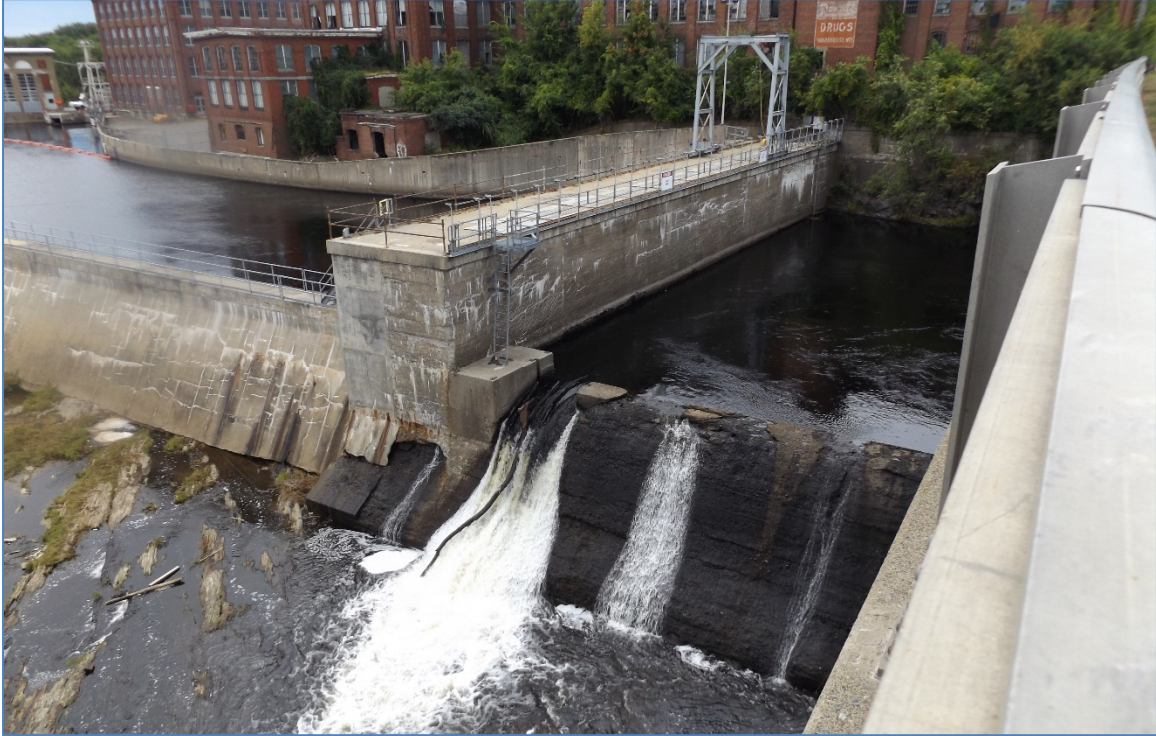
Figure 15 - Downstream Dam Spillway
