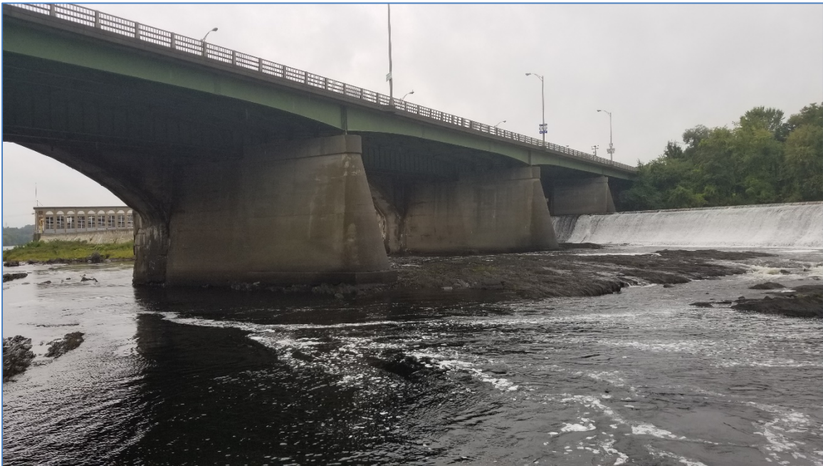
Figure 6 - Upstream Bridge Elevation Looking Southwest
