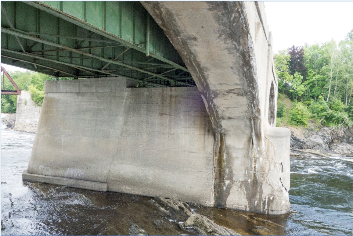
Figure 12 - East Pier Looking East
