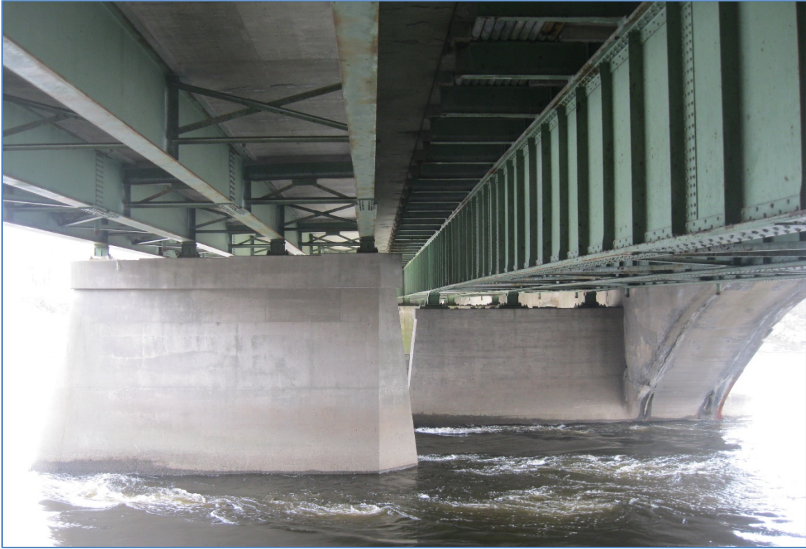
Figure 17 - West Piers, Looking East
