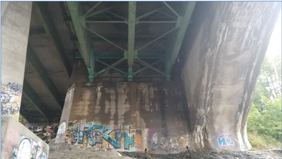
Figure 8 - Downstream East Abutment Looking East
