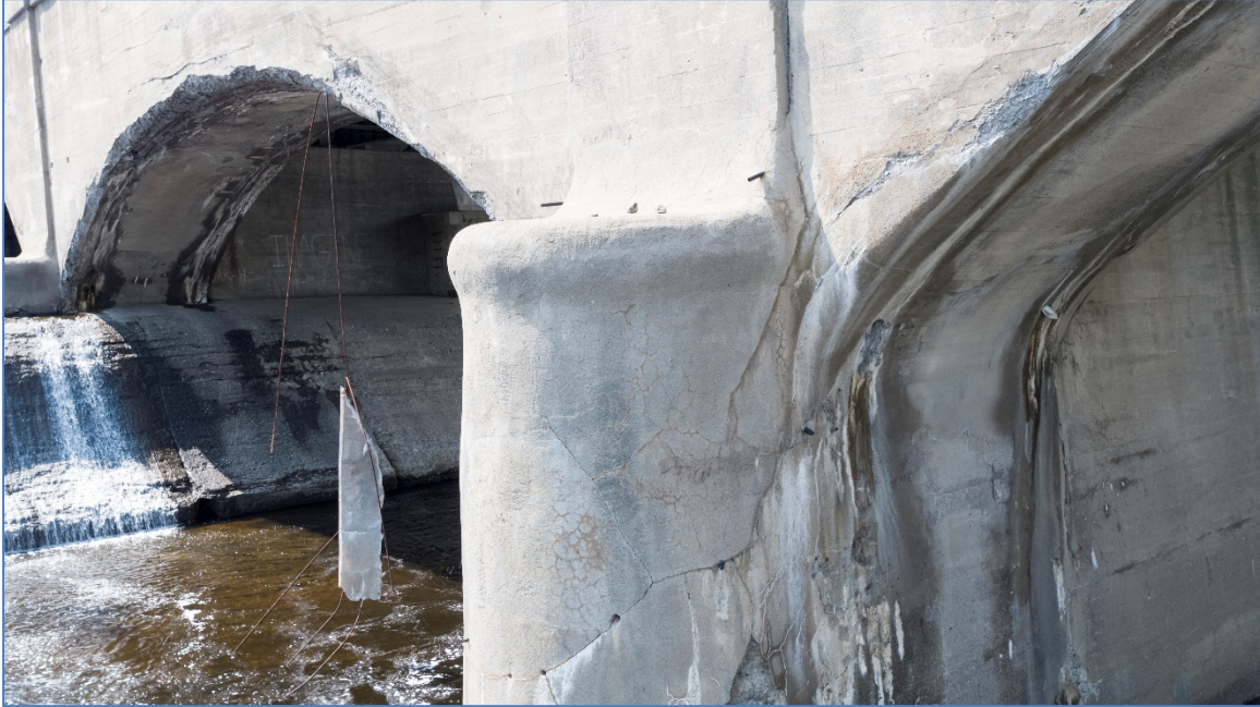
Figure 5 - Arch Condition Looking West
