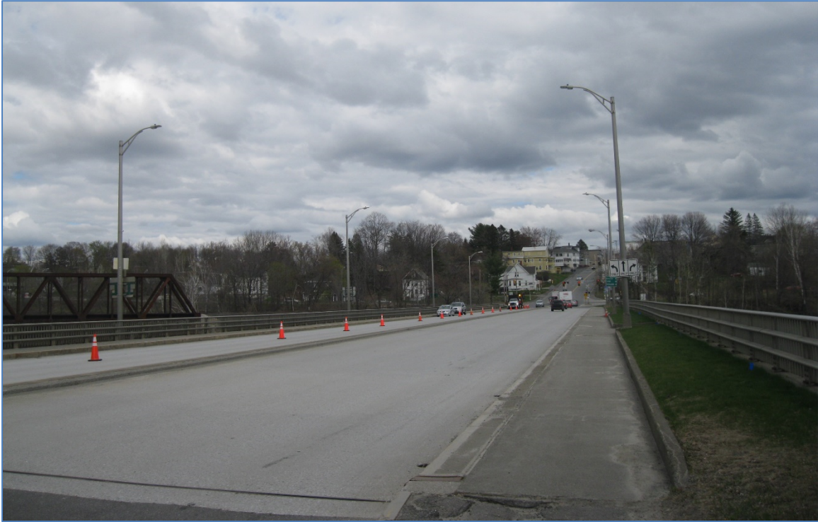
Figure 3 - Bridge Deck Looking East
