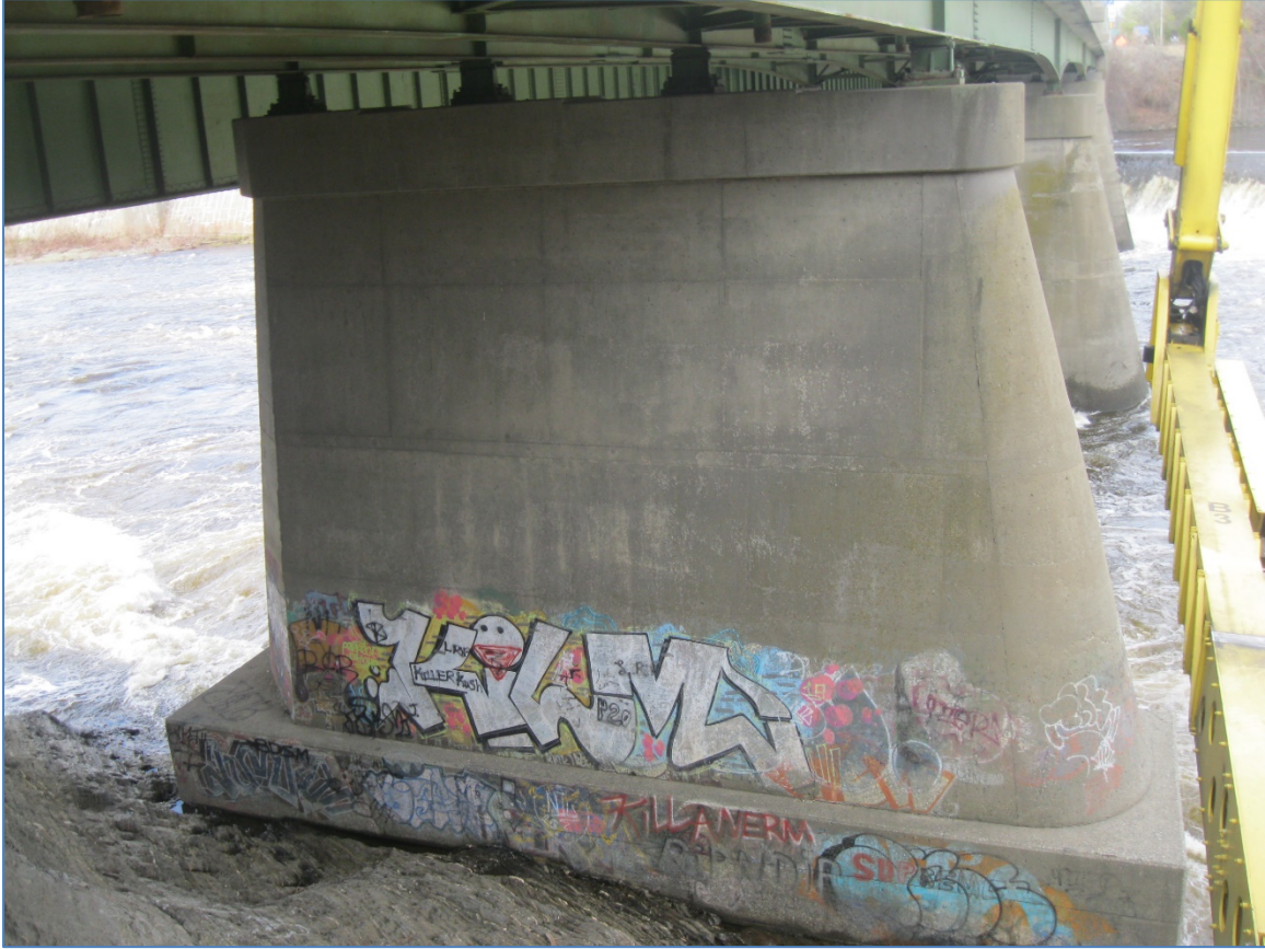
Figure 13 - Upstream East Pier Looking West
