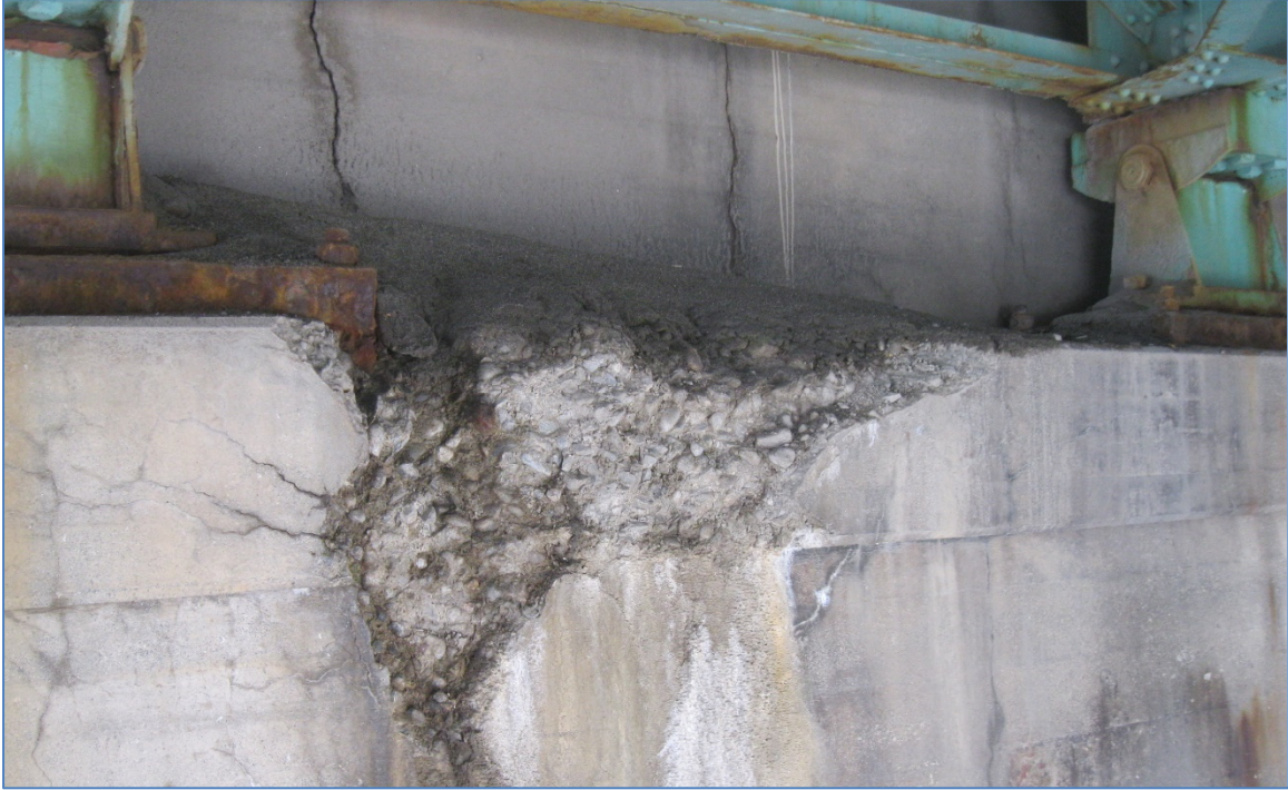
Figure 9 - East Abutment Seat
